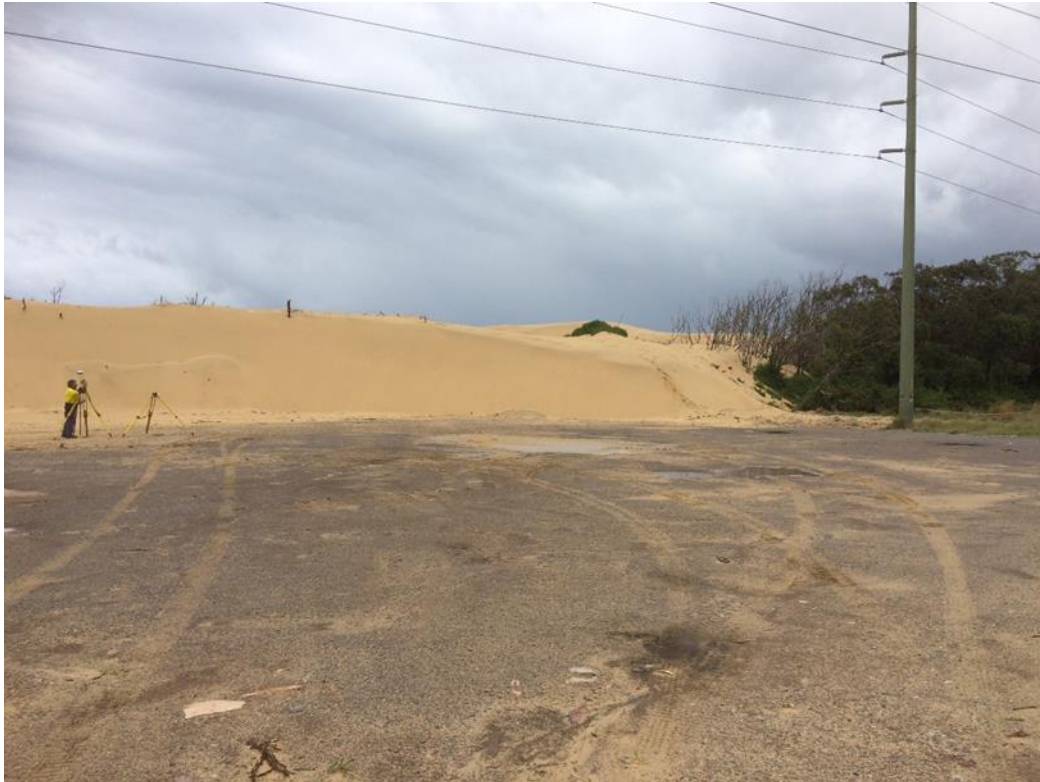
Plate 2-11: View South - West through Electricity Easement Following Emergency Removal of Sand Incursion Under Easement
